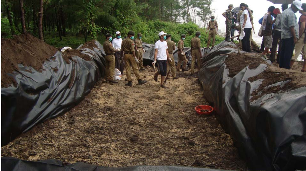
Pit Prepared for the bioremediation with working cadets and TERI
