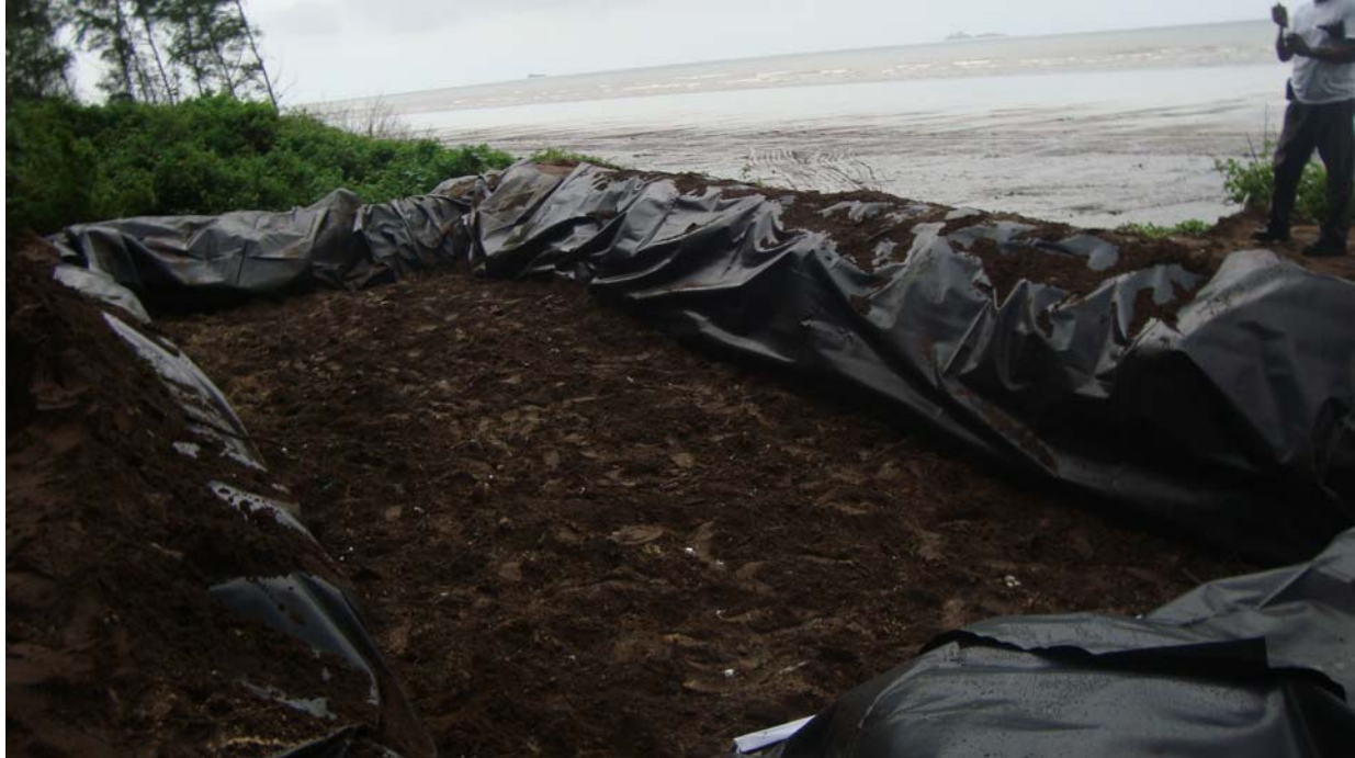
Pit after the completion of bioremediation.
