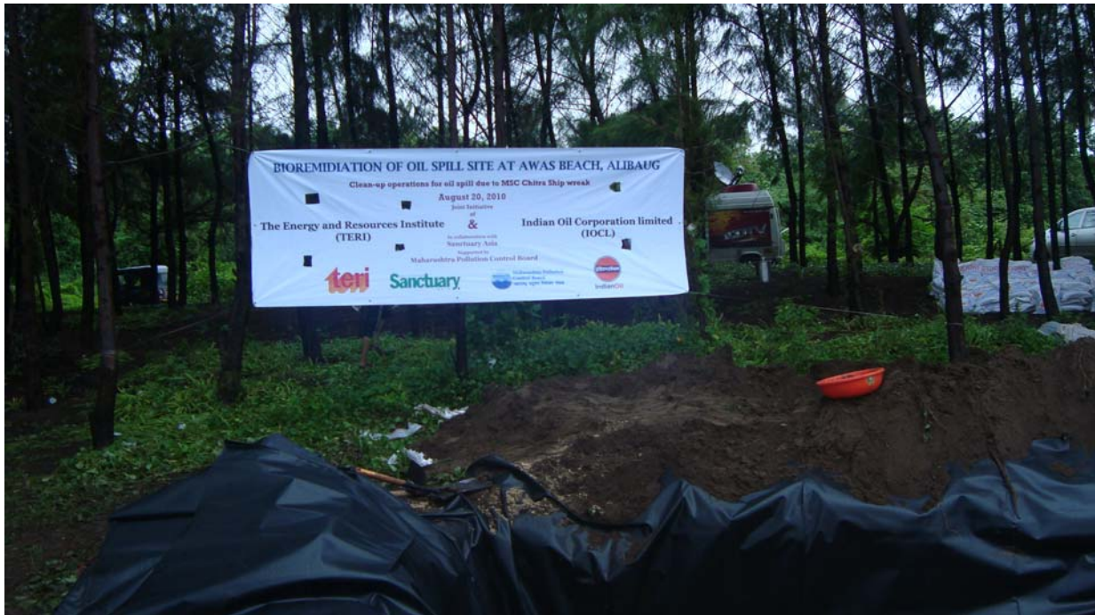
Site of pit
